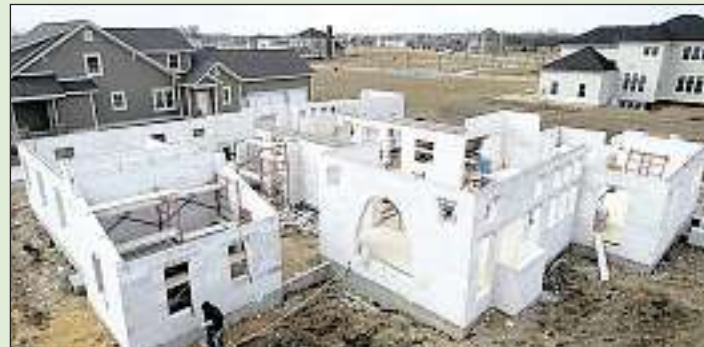
Autoclaved Aerated Concrete basic ingredients include sand, cement, lime, gypsum and water.
